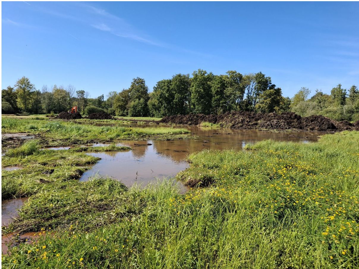
Peatland restoration works in Vorsdonkbos
