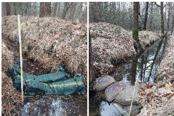
Sandbags as “weirs” installed to block off ditches in Breeven Site
