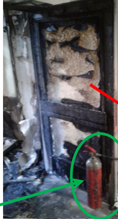
Fire door on side of flames
