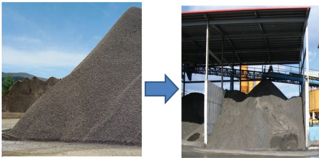
Figure 11. Non-protected stockpile (left) vs protected stockpile (right)
