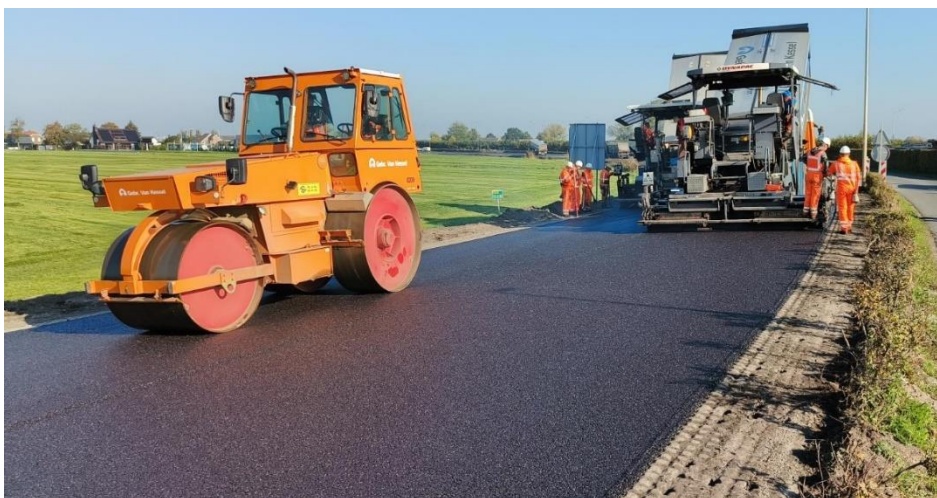
Figure 3. Application of biobased asphalt.
